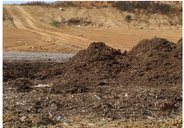
Step 2: Place Woodchips-Sludge Mix on Top of the Horse
