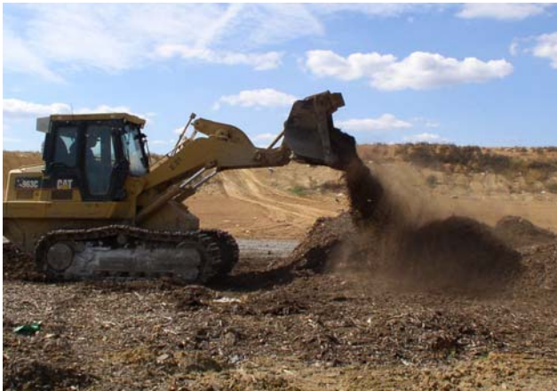
Step 3: Place Insulating Blanket on Top of the Mix
