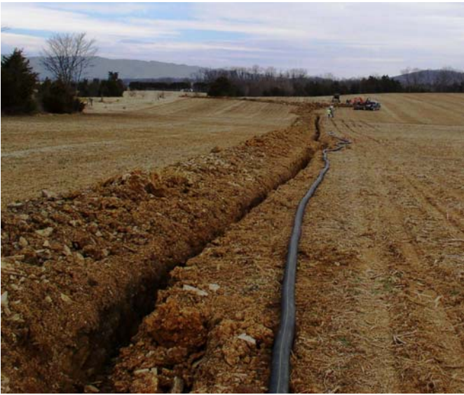
Installing a water line to supply water for livestock.
