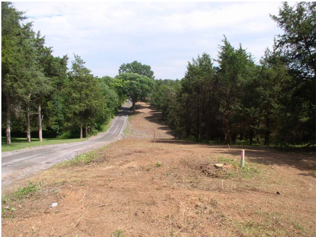
Clearing trees and fence construction along Teaberry Road.
